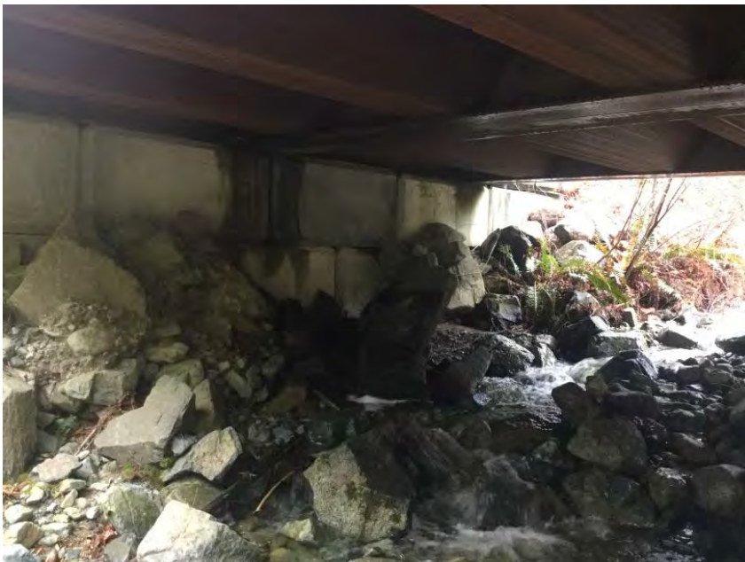
Right Bank Abutment when facing downstream
