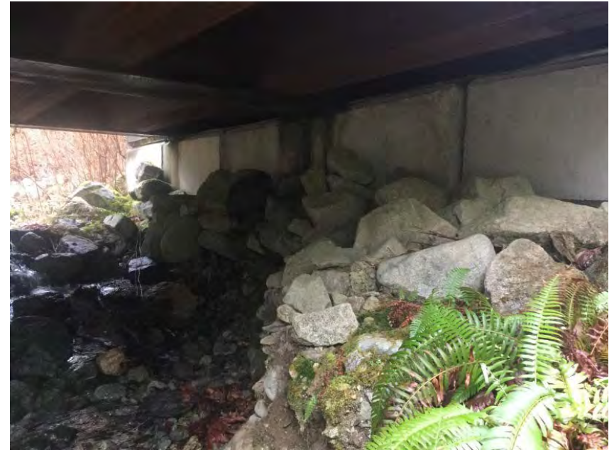
Left Bank Abutment when facing downstream
